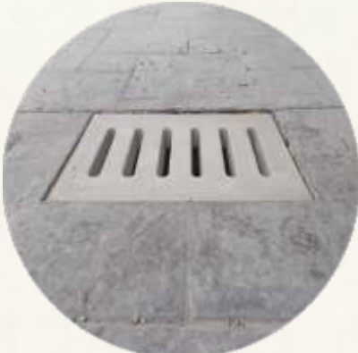
UNDER GROUND DRAINAGE & SEWER
